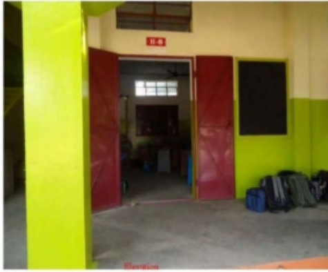
Polling Station Building Front View
