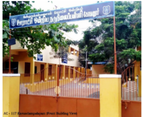
AC - 117 Koundampalayam (Front Building View)
