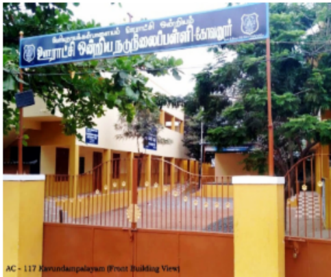
AC - 117 Koundampalayam (Front Building View)
