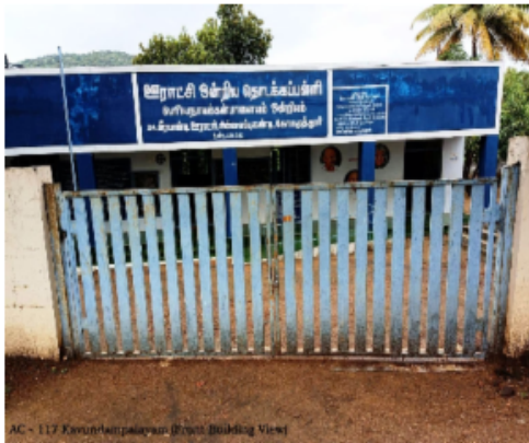
AC - 117 Kanurampalayam (Front Building View)
