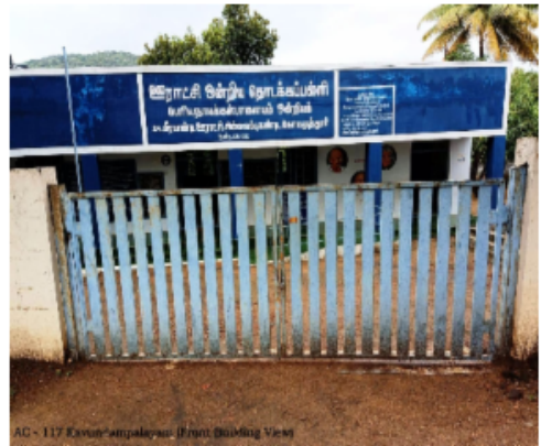
AC - 117 Kanurampalayam (Front Building View)
