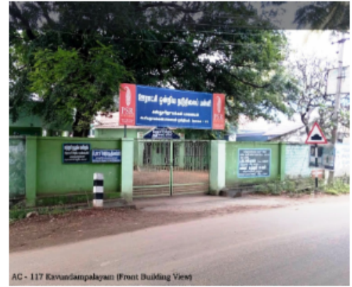
AC - 117 Kavundampalayam (Front Building View)
