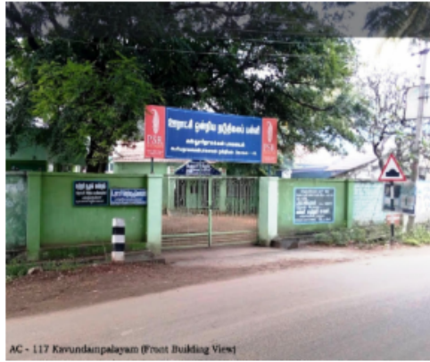
AC - 117 Kavundampalayam (Front Building View)
