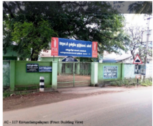
AC - 117 Kavundampalayam (Front Building View)
