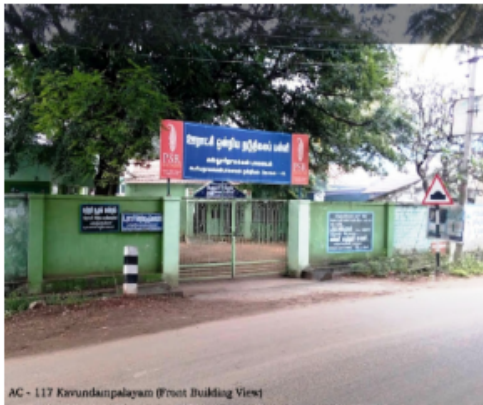
AC - 117 Kavundampalayam (Front Building View)
