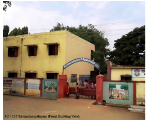
AC - 117 Karundampalayam (Front Building View)
