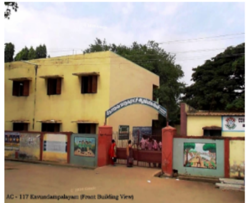
AC - 117 Karundampalayam (Front Building View)
