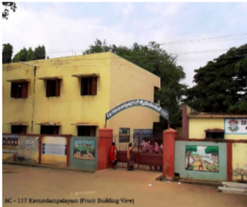
AC - 117 Karundampalayam (Front Building View)
