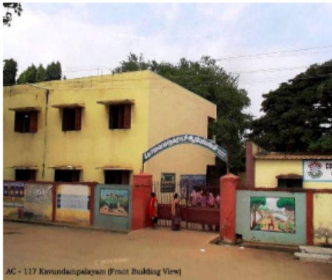
AC - 117 Karundampalayam (Front Building View)
