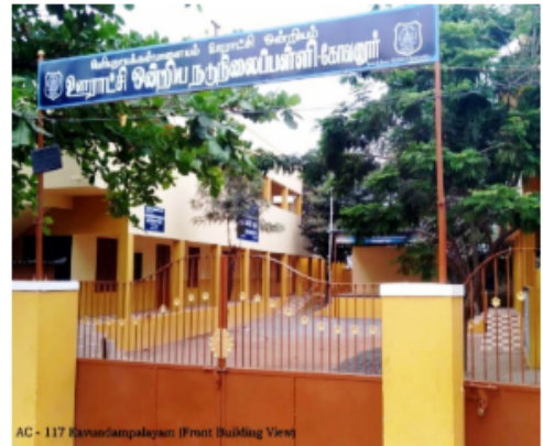
AC - 117 Koundampalayam (Front Building View)
