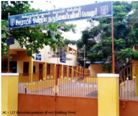
AC - 117 Koundampalayam (Front Building View)
