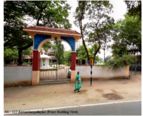
AC - 117 Karundampalayam (Front Building View)
