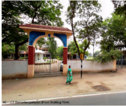
AC - 117 Karundampalayam (Front Building View)
