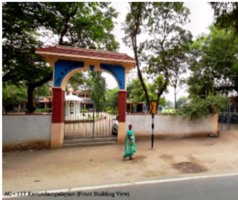
AC - 117 Karundampalayam (Front Building View)
