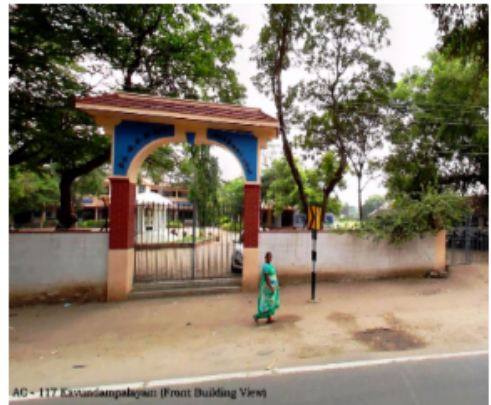
AC - 117 Karundampalayam (Front Building View)
