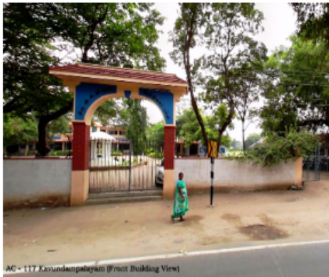
AC - 117 Karundampalayam (Front Building View)
