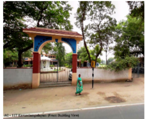
AC - 117 Karundampalayam (Front Building View)
