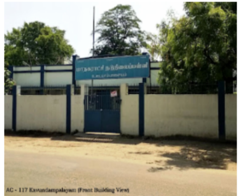
AC - 117 Kavundampalayam (Front Building View)
