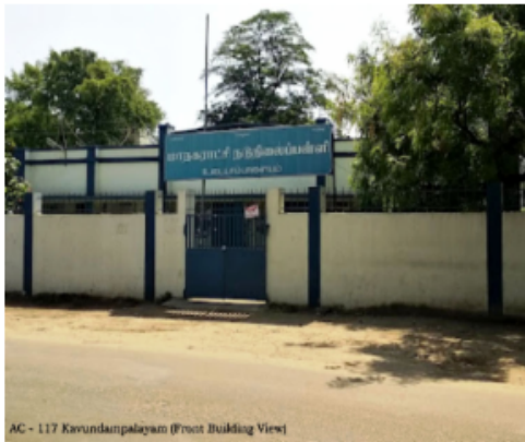
AC - 117 Kavundampalayam (Front Building View)
