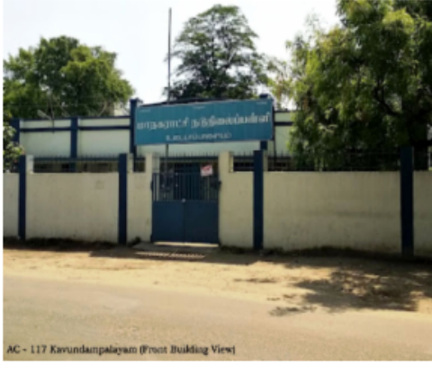
AC - 117 Kavundampalayam (Front Building View)
