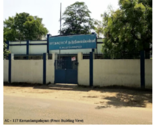
AC - 117 Kavundampalayam (Front Building View)
