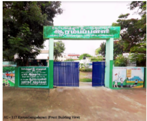
AC - 117 Karundampalayam (Front Building View)
