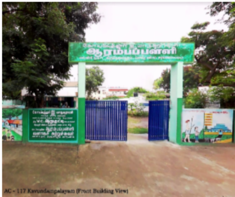
AC - 117 Karundampalayam (Front Building View)
