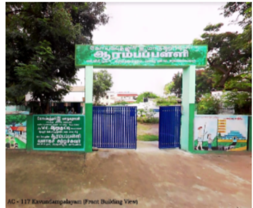
AC - 117 Karundampalayam (Front Building View)
