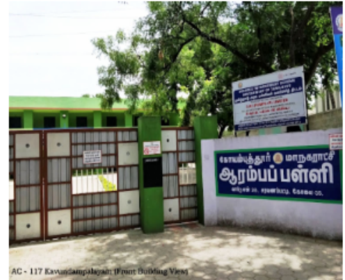
AC - 117 Karundampalayam Front Building View
