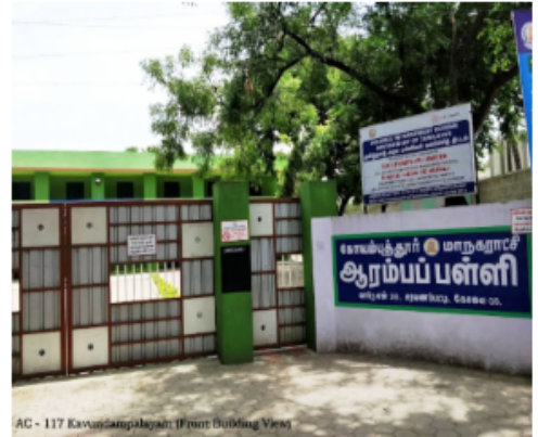
AC - 117 Karundampalayam Front Building View
