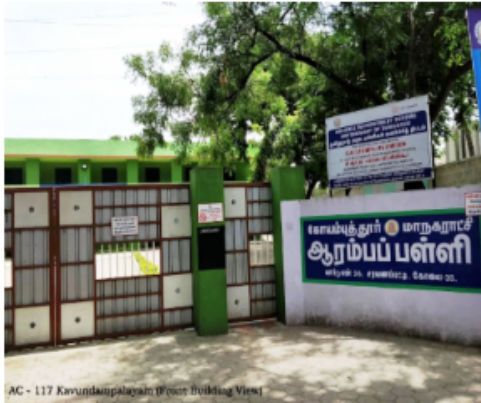
AC - 117 Karundampalayam Front Building View
