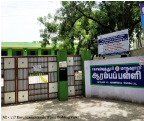
AC - 117 Kavayitriccummandam Front Building View
