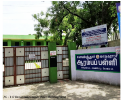
AC - 117 Kavayampalayam Front Building View
