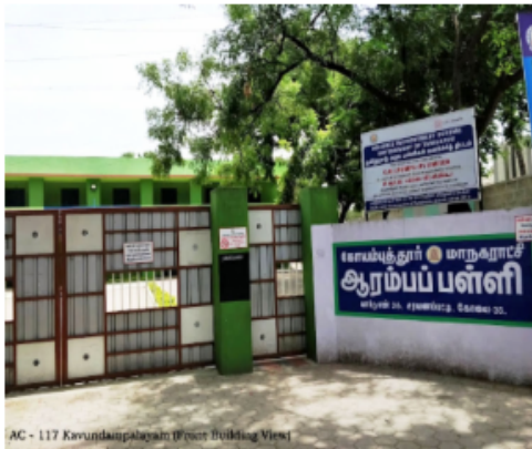
AC - 117 Kavayampalayam Front Building View
