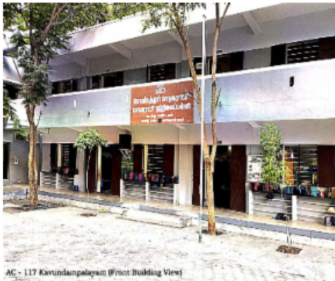
AC - 117 Kivundampalayam (Front Building View)
