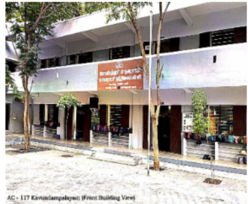
AC - 117 Kivundampalayam (Front Building View)
