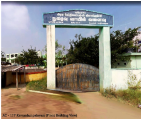
AC - 117 Karundampalayam (Front Building View)
