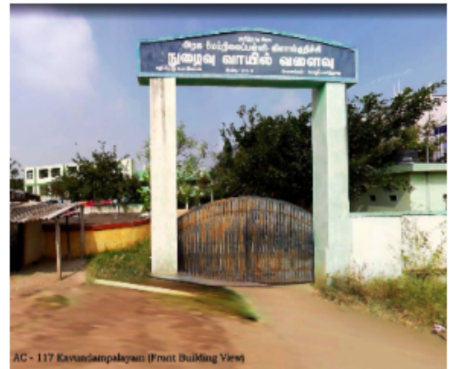
AC - 117 Karundampalayam (Front Building View)
