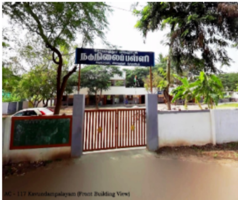
PS - 117, Koundampalayam (Front Building View)
