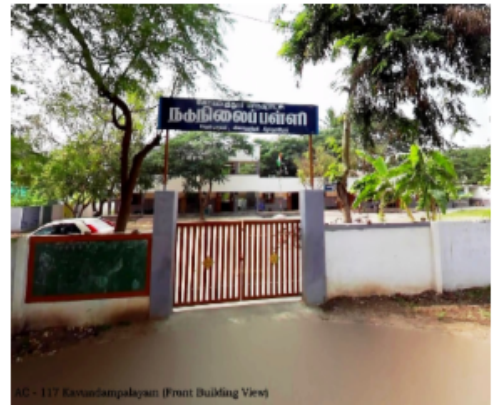
PS - 117, Koundampalayam (Front Building View)
