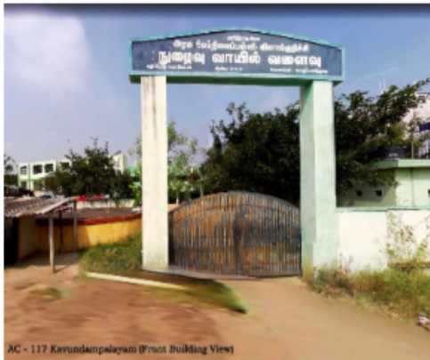
AC - 117 Karundampalayam (Front Building View)
