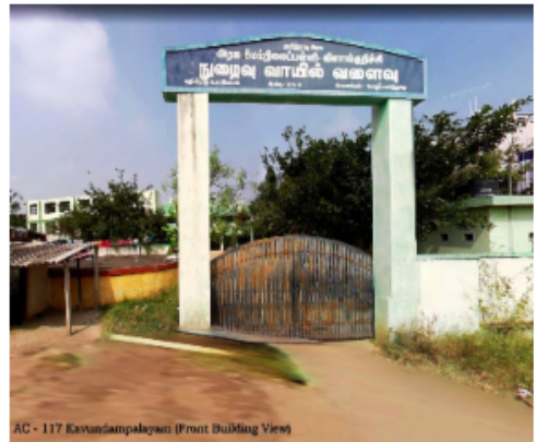
AC - 117 Karundampalayam (Front Building View)
