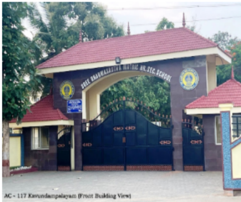
AC - 117 Kavundampalayam (Front Building View)
