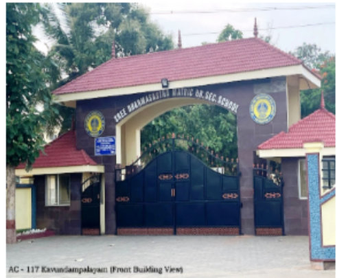
AC - 117 Kavundampalayam (Front Building View)
