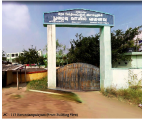
AC - 117 Karundampalayam (Front Building View)
