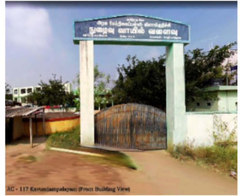
AC - 117 Karundampalayam (Front Building View)
