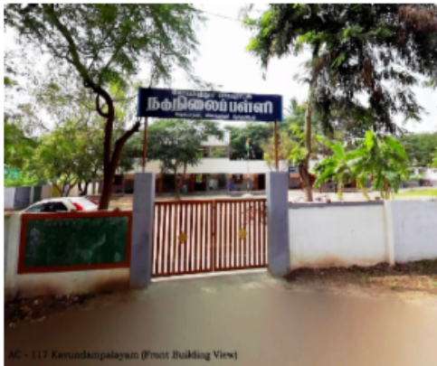
PS - 117, Koundampalayam (Front Building View)
