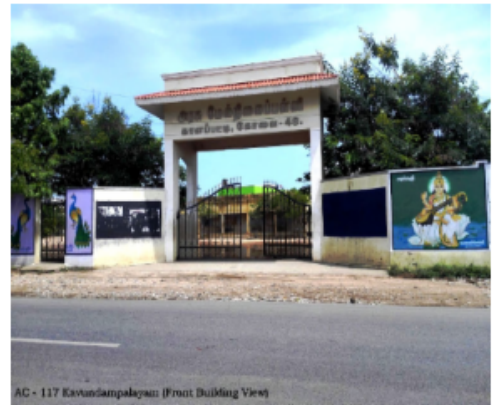
AC - 117 Kavundampalayam (Front Building View)
