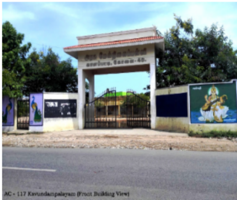
AC - 117 Kavundampalayam (Front Building View)
