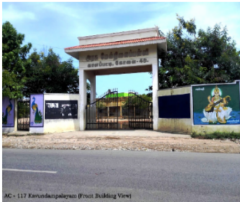
AC - 117 Kavundampalayam (Front Building View)
