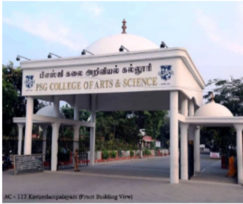
AC - 117 Karundampalayam (Front Building View)
