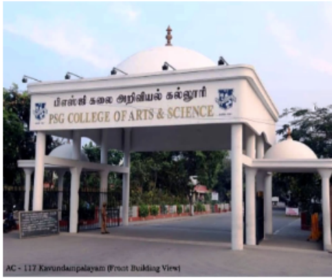
AC - 117 Karundampalayam (Front Building View)
