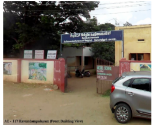
AC - 117 Kavundampalayam (Front Building View)
