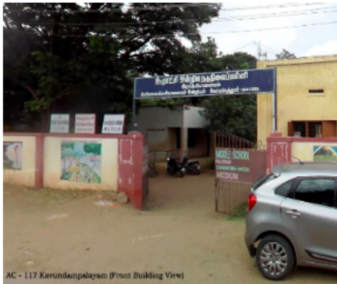
AC - 117 Kavundampalayam (Front Building View)
