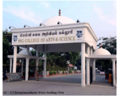
AC - 117 Karundampalayam (Front Building View)
