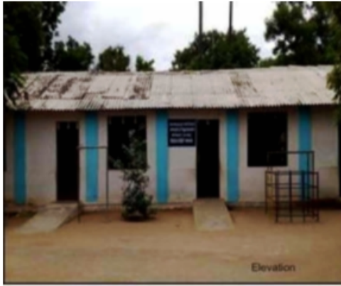
Polling Station Building Front View
