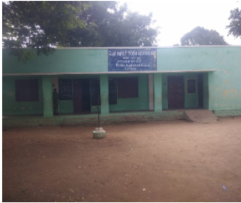
Polling Station Building Front View
