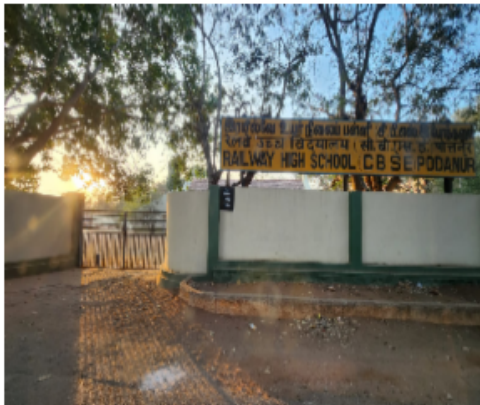
Polling Station Building Front View
