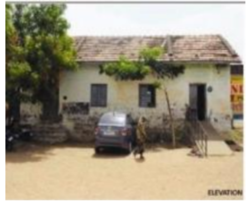
Polling Station Front View
