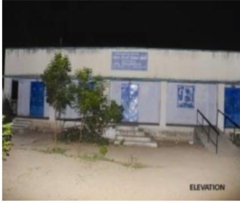
Polling Station Building Front View
