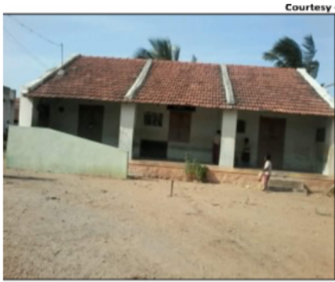
Polling Station Building Front View
