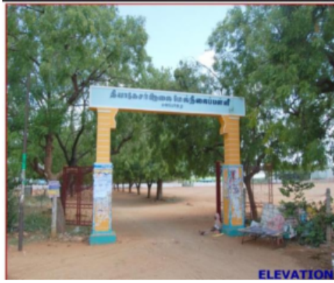
Polling Station Building Front View
