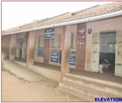
Polling Station Building Front View
