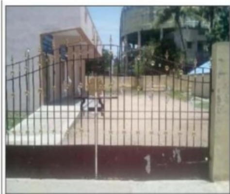
Polling Station Building Front View
