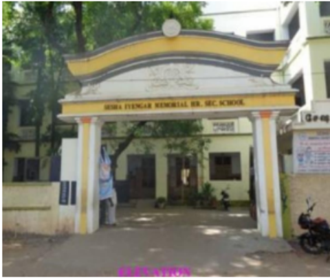
Polling Station Building Front View
