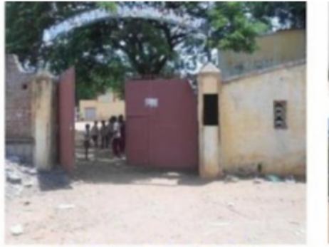
FRONT VIEW -( MAIN ENTRY )
