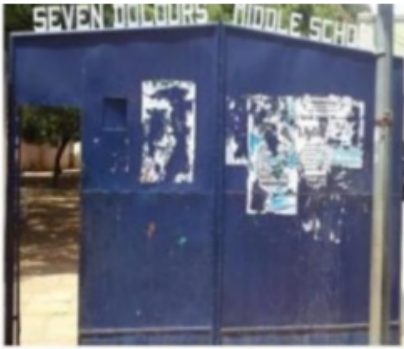
FRONT VIEW - ( MAIN ENTRY )
