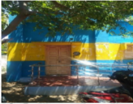
Polling Station Building Front View
