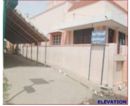
Polling Station Front View
