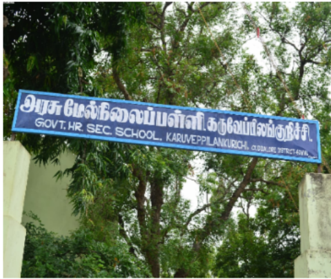
Polling Station Building Front View
