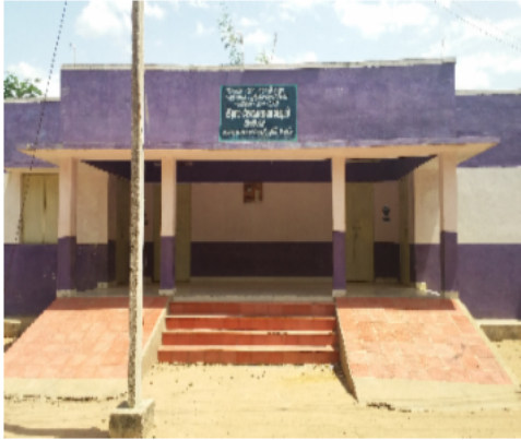
Polling Station Building Front View
