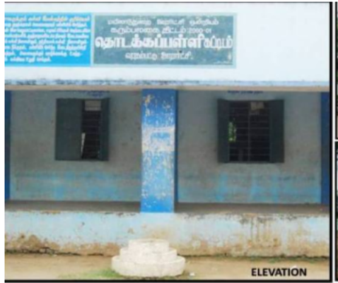
Polling Station Building Front View
